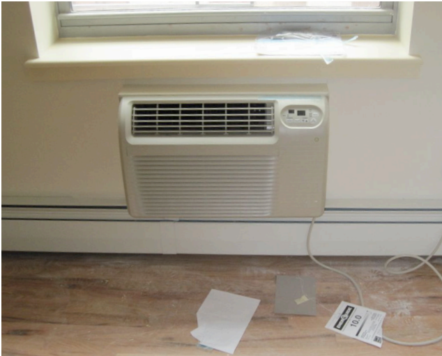
Fig. 4: Sleeve with AC installed
