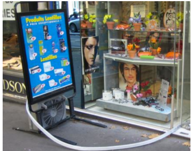
Fig. 20: “Packaged-Split” Installation in Europe
