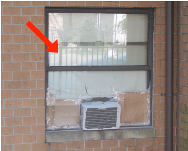
Fig. 3: Bad double-hung window installation
