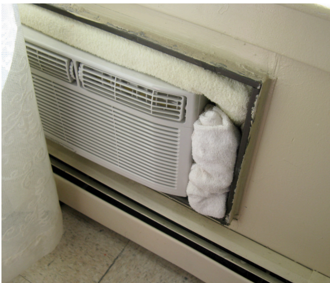
Fig. 7: Window AC installed in a sleeve
