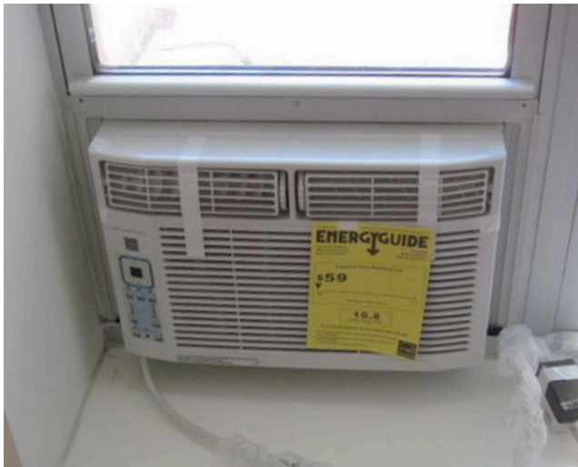
Fig. 2: Good double-hung window installation
