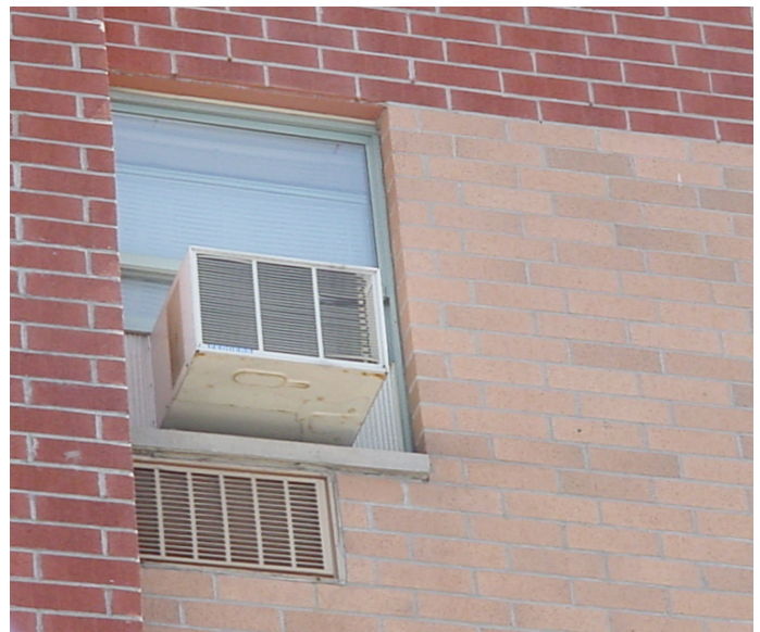
Fig. 8: Window AC above sleeve
