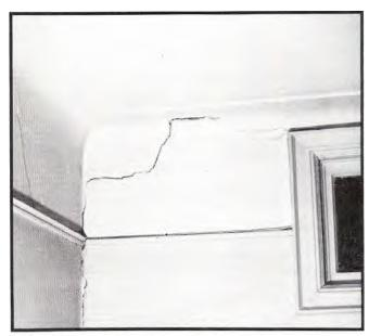
Settlement cracks to be patch plasteredand taped.
