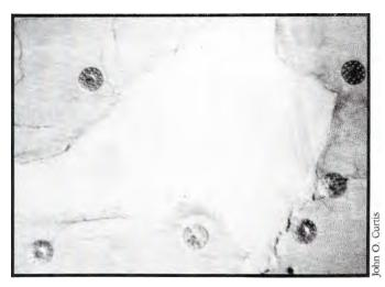
Washers secure the remaining old plaster around a hole that has been patched.
