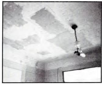
When large chunks of plaster are missing, drywall patches can he used as a base.
