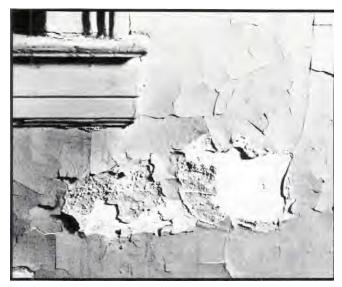
Paint and plaster failure from water penetration.
