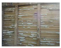
Prior to carrying out remedial work, buildings must be checked for safe entry and working conditions and structural adequacy. Detailed investigation needs to be carried out to establish the extent of damage to the structure and linings. Buildings must be returned to plumb and level before starting work on internal linings.
